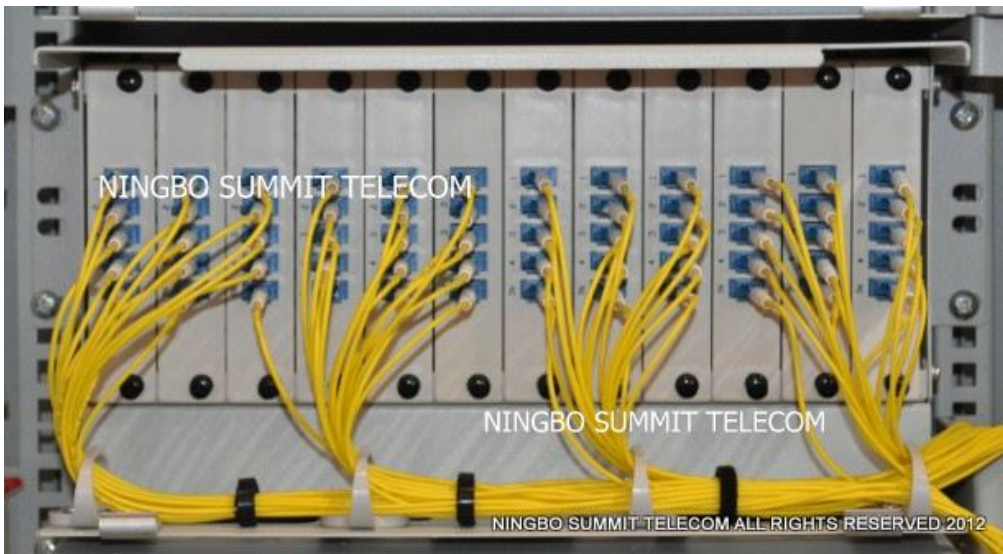
Splice Tray for go out fiber splicing, and fiber storage tray.
