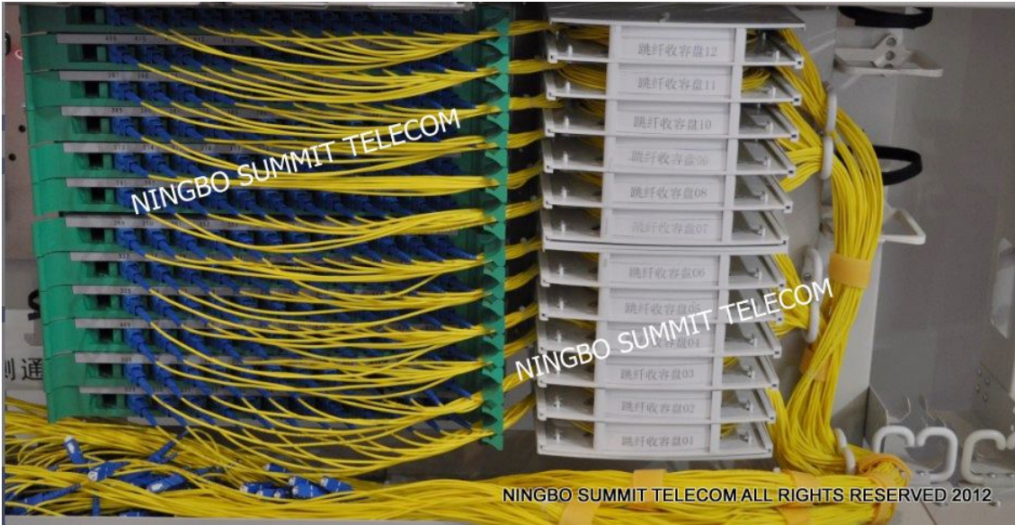
Pacth Tray on right side for fiber patching and termination.
