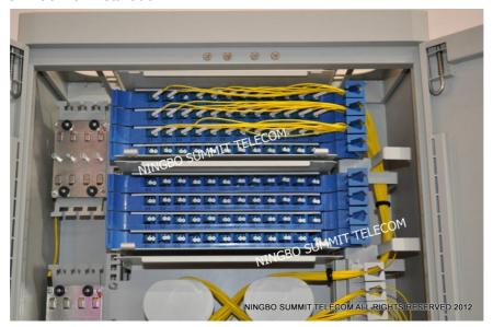
Could install PLC optical splitter for capacity enlarging.
