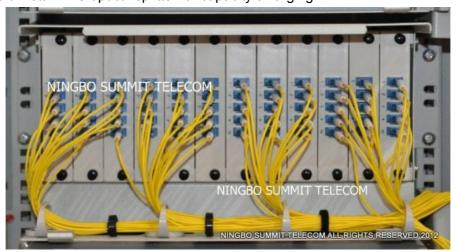
Splice tray for going out fiber splicing, storage tray for fiber storage, and there also are special management rings and ways so that makes fiber management clearer and trimer.
